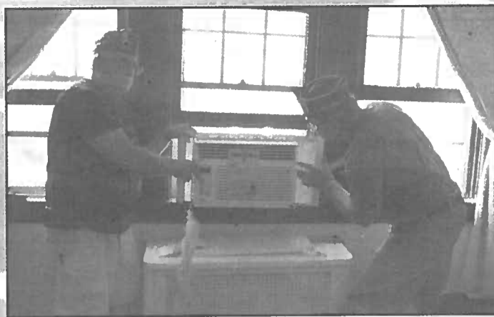
Post 917 members Frank Russo (left) and George Cusick install an air conditioner for a needy veteran.
